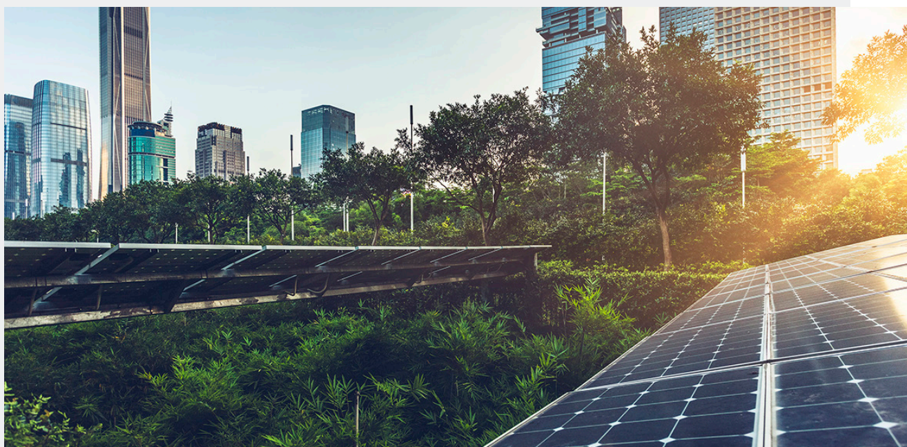
Rooftop solar installation, Shenzhen China. (Photo by aaaaimages / Getty Images).
