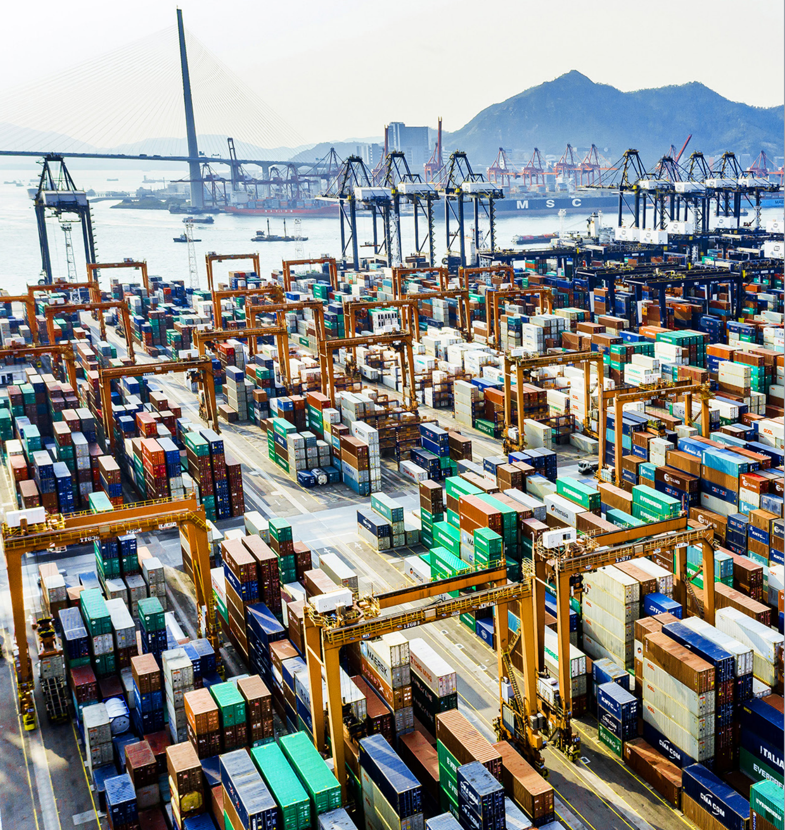
Container terminal, Hong Kong. (Photo by Chunyip Wong / iStock).
